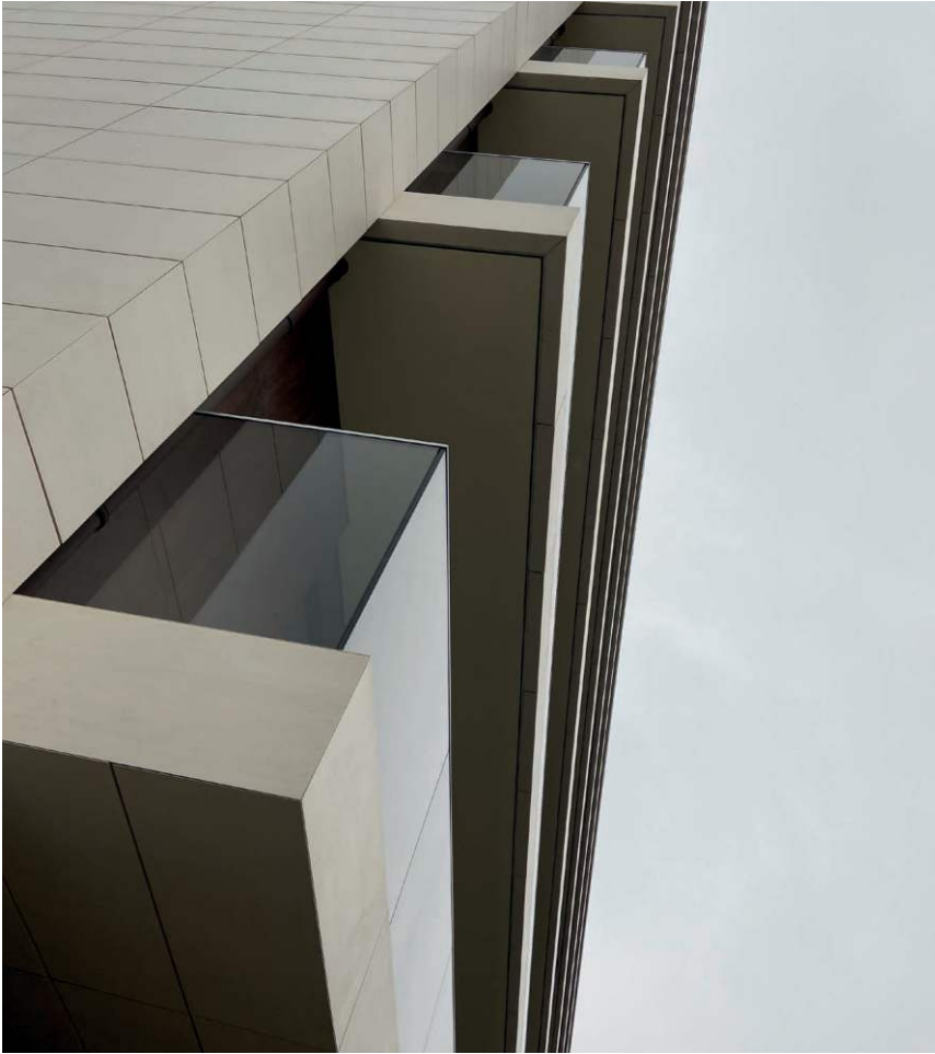
PORTUGAL - GAIA FLATS RESIDENTIAL BUILDING
